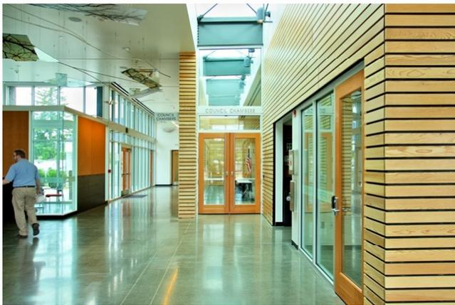
A linear skylight in the Large Meeting Room/Council Chambers extends into an adjacent Lobby and Gallery space, providing daylight illumination at areas that have no access to perimeter glazing. All ambient electric light sources are off in this image.
